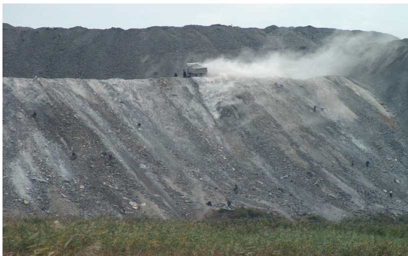
Fig. 2 – Unloading face for the industrial wastes.
